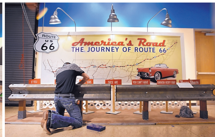
Exhibits technician Ryan Painter installs a guardrail for the National Museum of Nuclear Science and History.
