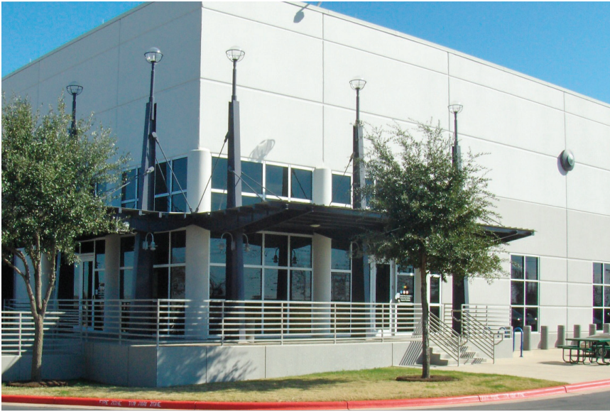
One of two data centers Waste Management operates.
