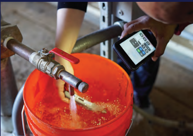
Sensors provide real-time conditions
