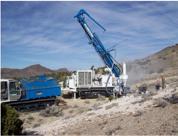
Drilling at Reveille
