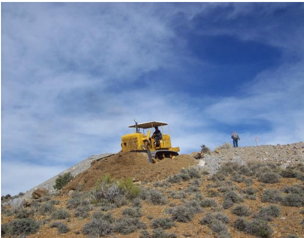
Building Road for Drilling
